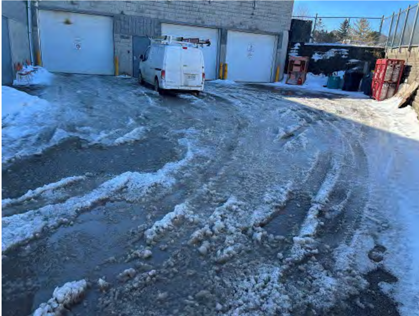
Rear ramp GIP – due to Ice Resurfacer dumping outside tracking water and unsandable
