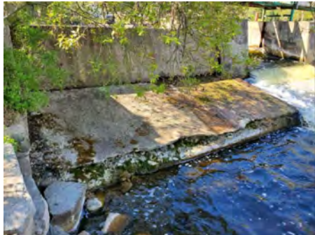
East Concrete Apron
