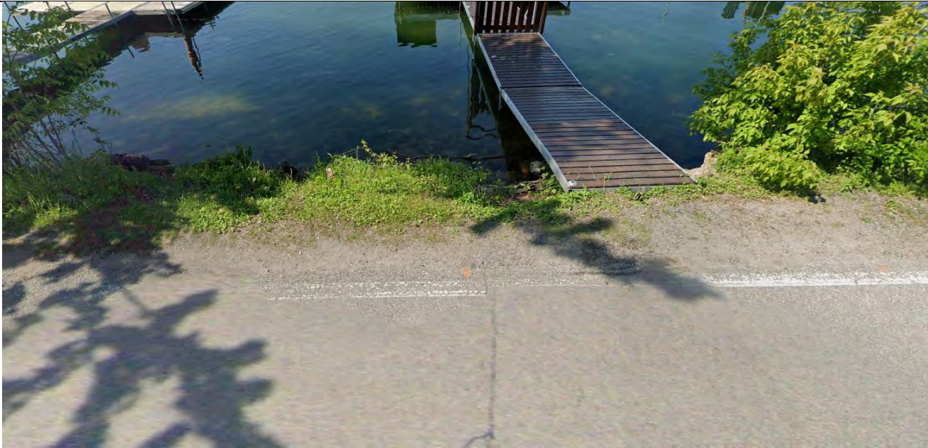
Lake Drive North (Area of Concern – Proximity of Shoreline)
