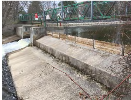
Downstream Looking South
