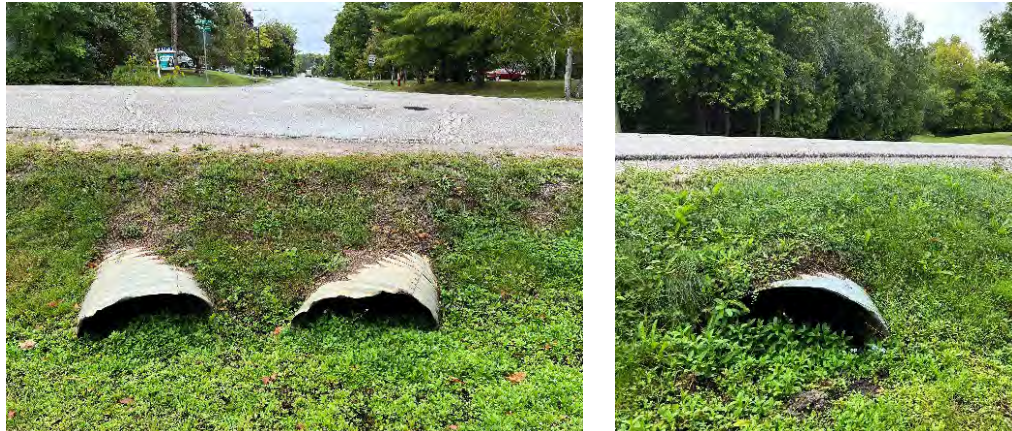
Figure 2: Cedar Grove Road transverse culvert
