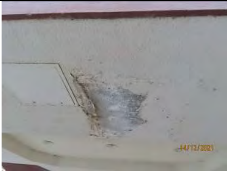
Damaged soffit and flat roofing – Pefferlaw Lions Hall Canopy
