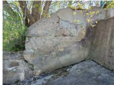
Downstream East Retaining Wall
